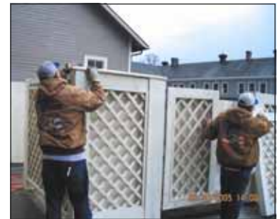
Constructing a trash enclosure at West Barracks
