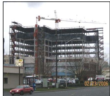
Commercial Construction Southwest WA Medical Center Expansion
