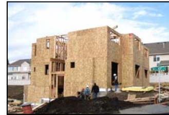
Residential Construction-43rd ST
