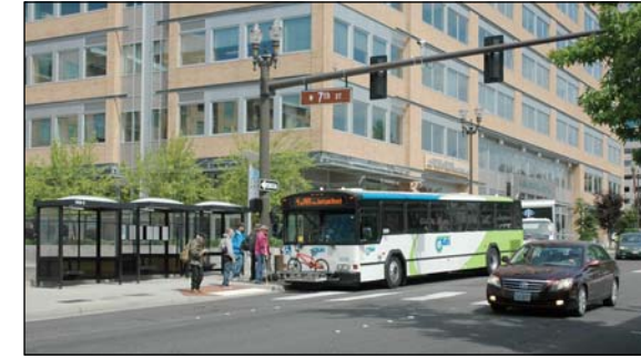
C-Tran's service modification removed buses from Main Street and created several convenient new bus stops in the downtown area.
