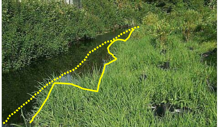
The solid line shows extensive damage caused by nutria in the Burnt Bridge Creek Greenway. Dotted line is original creek bank.
