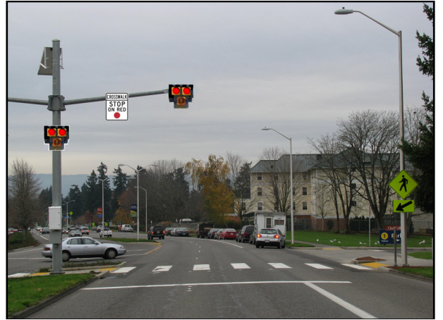
Future overhead, pedestrian hybrid signal. (Clark College crossing on Fort Vancouver Way)
