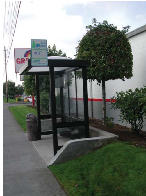
Figure 28 | Side wall of Grocery Outlet along Fourth Plain Boulevard 4P Policy 2. Create design standards for public and private development that emphasize building local diversity and attractive boulevard character. Tie pulse points together with streetscape improvements, composed of distinctive treatments that are appropriate to adjacent uses and reflect neighborhood character.
