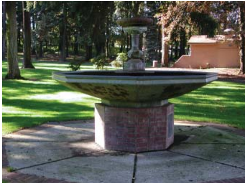
Figure 13 | Waterworks Park 4P Action Item 18. Work with Vancouver-Clark Parks and Recreation and the Vancouver Police Department to explore ways of improving user and facility security and safety at Waterworks Park and Evergreen Park after dark, such as better lighting near Fourth Plain Boulevard and raising using tree canopy or thinning of trees directly adjacent to discourages use of the park after closing time (dusk) for illegal activities. Consistent police enforcement of park hours (7am to dusk) is encouraged (see Fourth Plain Plan, Goals and Policies, page 51).
