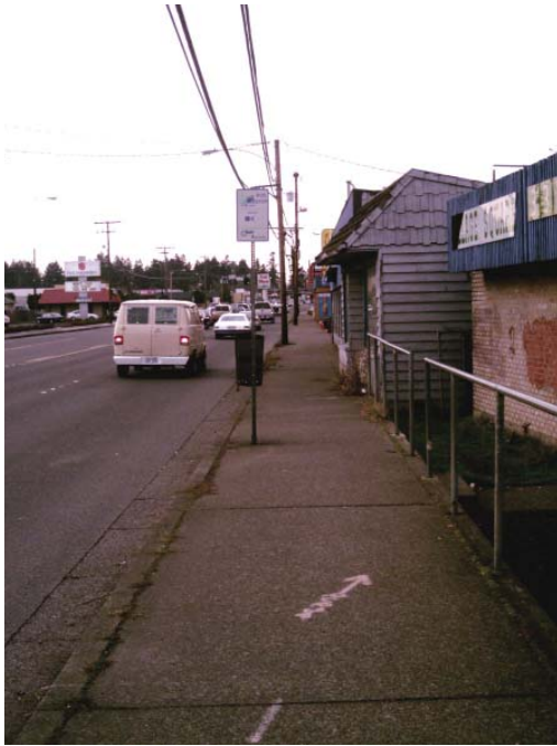
Figure 11 | Narrow sidewalk along Fourth Plain Boulevard 4P Action Item 26. Establish minimum 10- to 12-foot-wide sidewalks on Fourth Plain Boulevard. Explore building continuous sidewalks with limited curb cuts, street trees, landscaping and/or street furnishing zone between sidewalk and road, prominent transit features, bike lanes, and median diverters (see Fourth Plain Plan, Goals and Policies, page 53).
