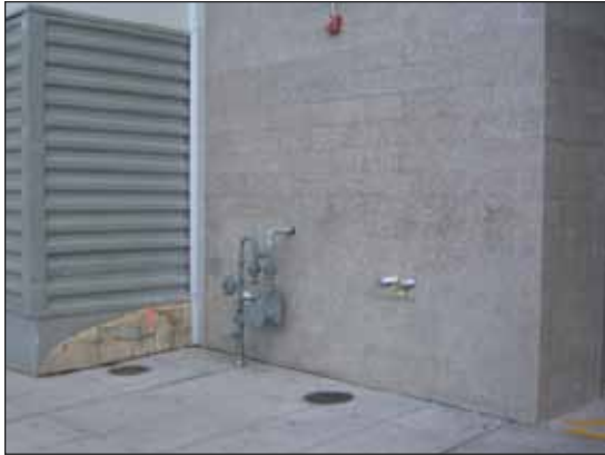
Figure 22. Avoid exposed utility meters placed directly on the sidewalk.
