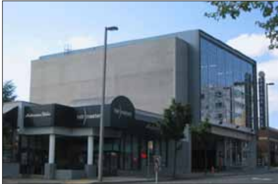
Figure 44. Blank, visible, and plain CMU fire walls like this are prohibited. Such buildings should incorporate patterns of different CMU colors or textures or different materials to add visual interest to such visible firewalls.
