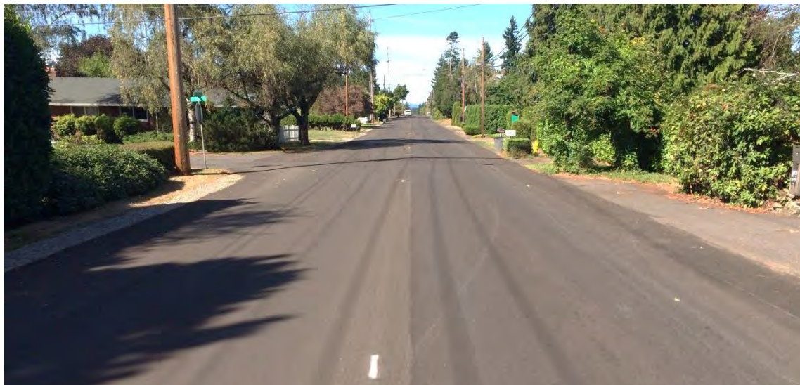
Photo 40. Kauffman/Lincoln Avenue Condition 4: 39th Street to Bernie Road
