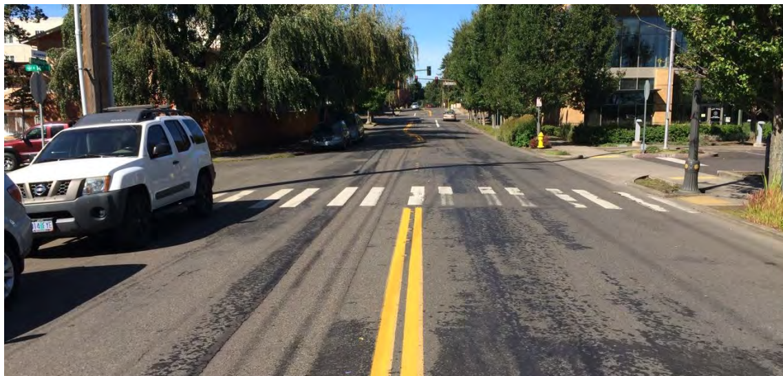
Photo 38. Kauffman/Lincoln Avenue Condition 2: 13th Street to Fourth Plain Boulevard
