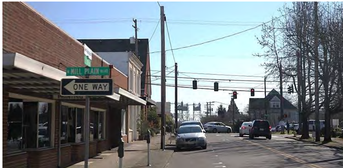
Photo 34. Columbia Street Condition 4: Between 13th and 16th Streets
