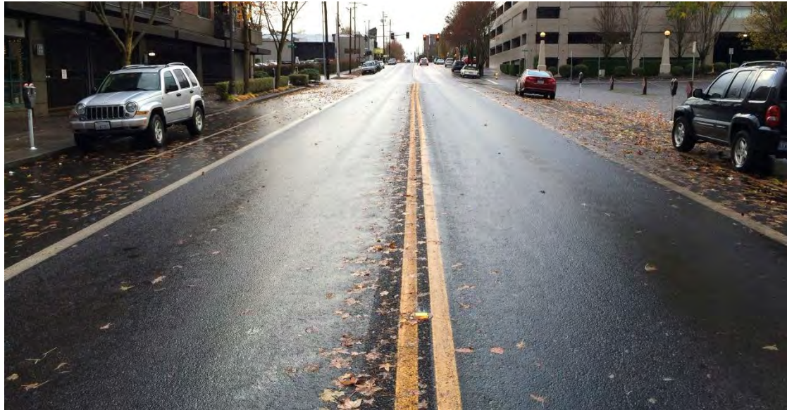
Photo 33. Columbia Street Condition 3: Between 8th and 12th Streets
