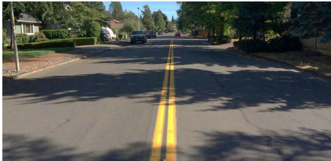
Photo 41. Kaufmann/Lincoln Avenue Condition 5: Bernie Road
