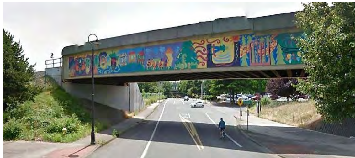
Photo 31. Columbia Street Condition 1: South of 5th Street
