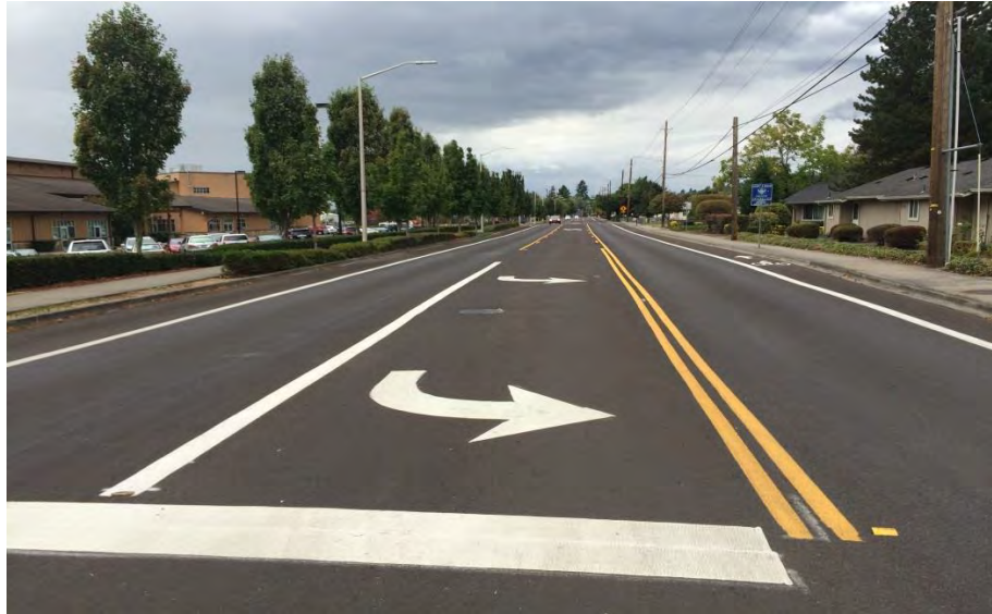
Photo 25. Fruit Valley Road Condition 1: Fruit Valley Elementary School
