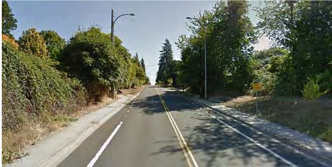
Photo 21. 39th Street Condition 2: East of Railroad Bridge
