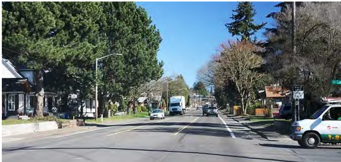
Photo 18. Fourth Plain Condition 2: Between Railroad Bridge and Columbia Street
