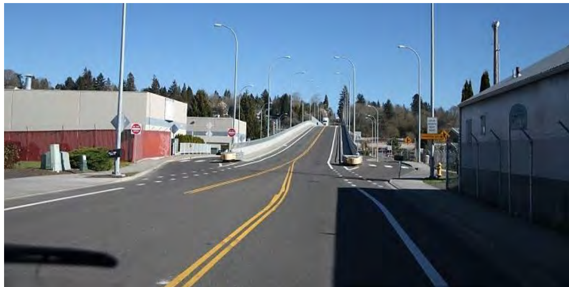
Photo 20. 39th Street Condition 1: West of Railroad Bridge
