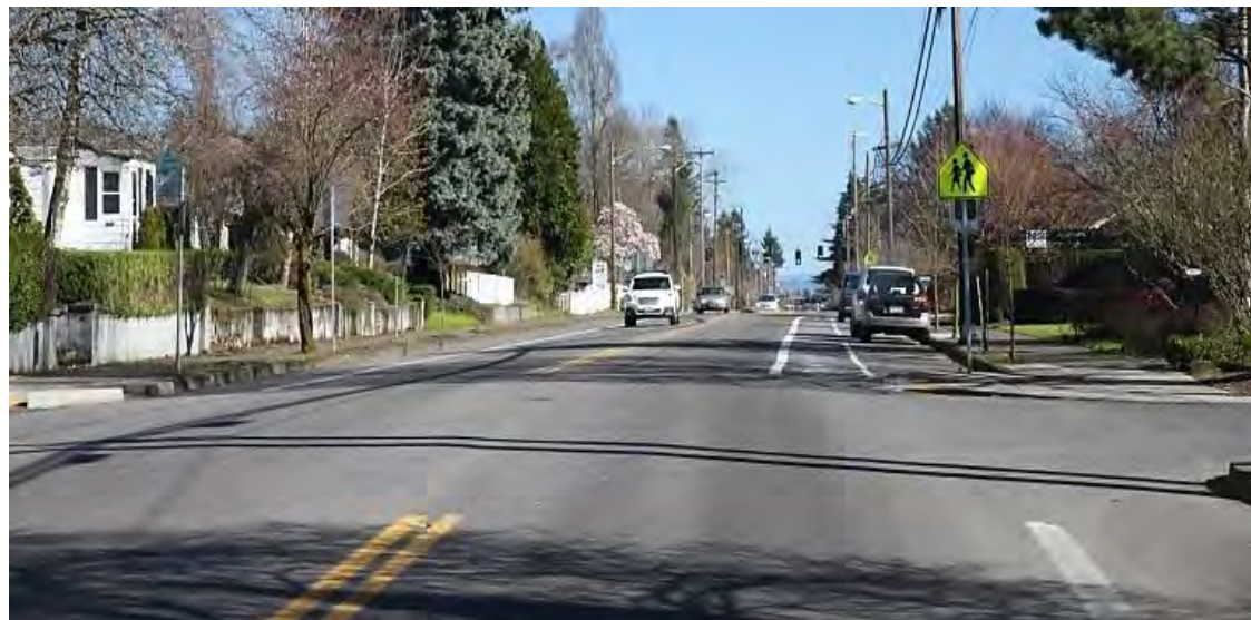
Photo 22. 39th Street Condition 3: Between Lincoln Avenue and Columbia Street
