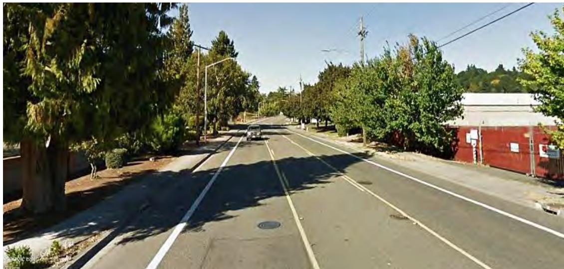
Photo 26. Fruit Valley Road Condition 2: Between 37th Street and 61st Street
