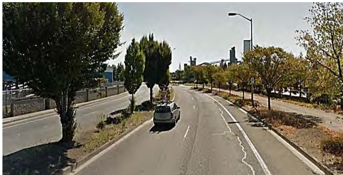
Photo 14. Mill Plain Condition 1: West of Railroad Bridge
