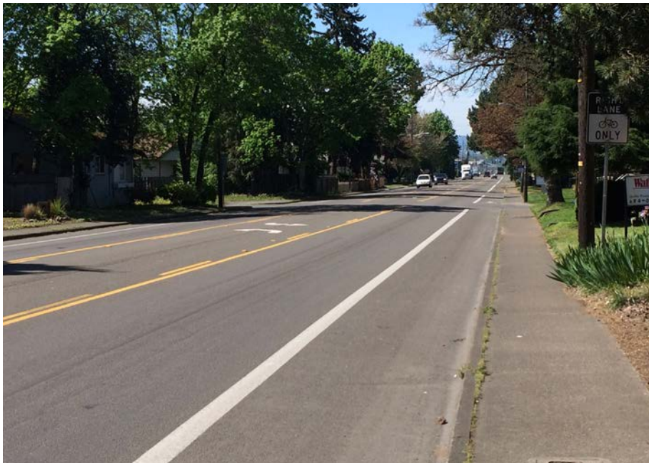
There is nearly 2000 linear feet between marked pedestrian crossings of Fourth Plain Blvd. between Columbia St. and Kauffman Ave.
