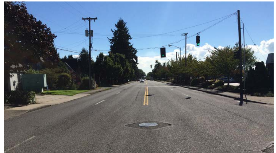
Upper Main's four-lane design and wide travel lanes encourages high speeds and diversion traffic from I-5
