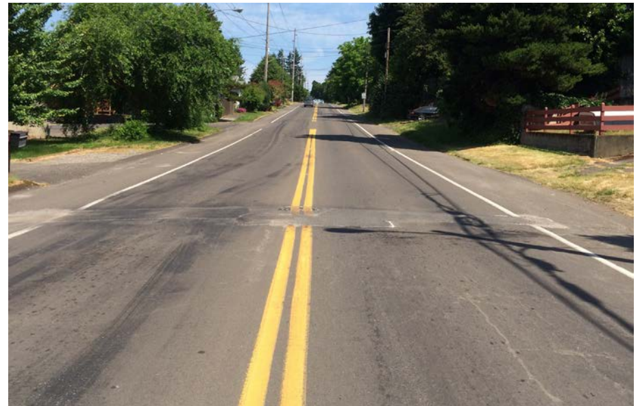
Lincoln Avenue is the only arterial on the westside without sidewalks
