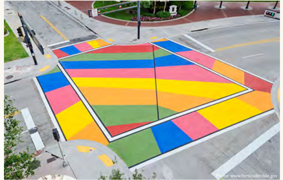
Drivers tend to slow down on approach because the paint signals the presence of pedestrians
