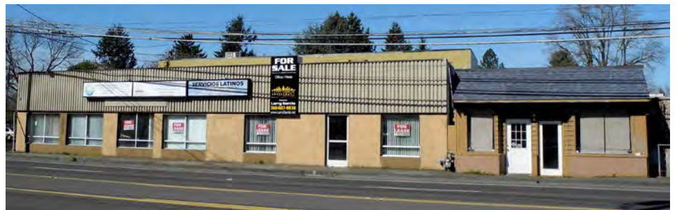
A vacant space that may benefit from a minor storefront improvement or adaptive reuse assistance
