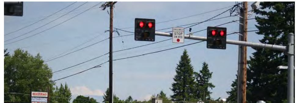
Community members feel that many cars do not notice the HAWK pedestrian signals
