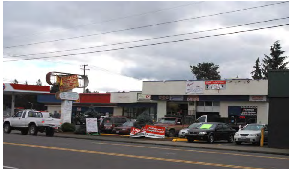
Many buildings are in fair or poor condition
