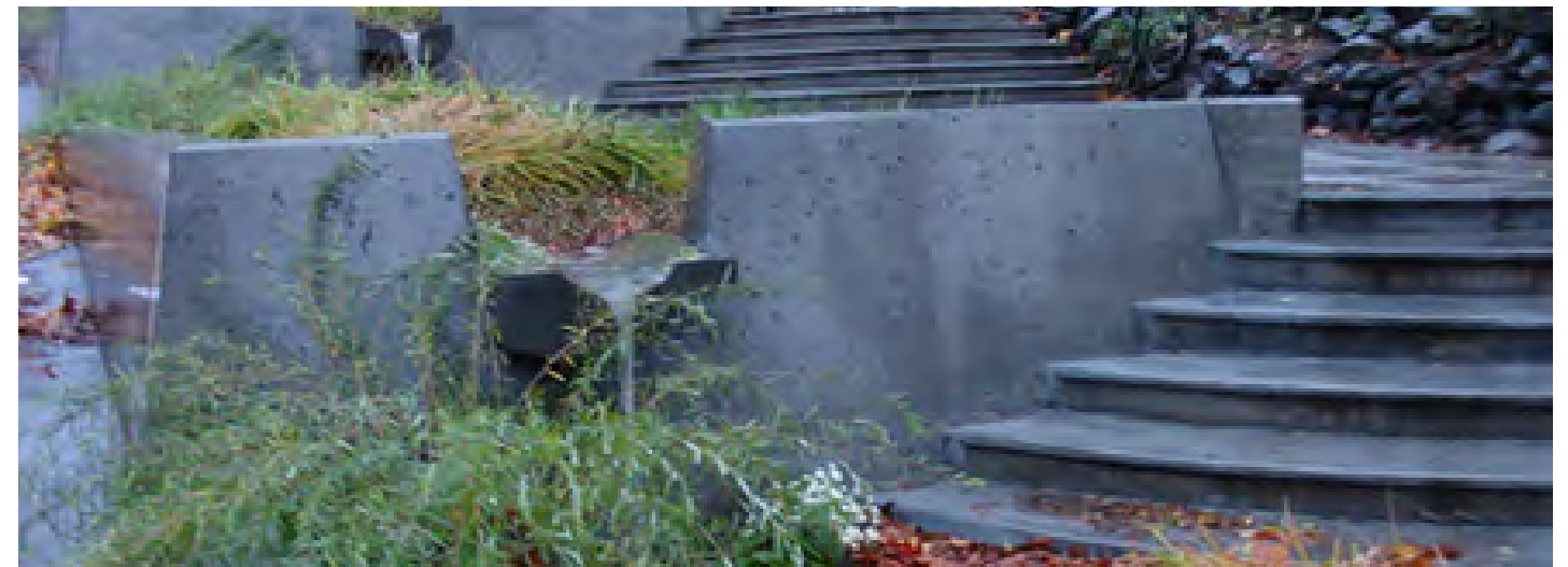
Integrated Stormwater Management Systems
