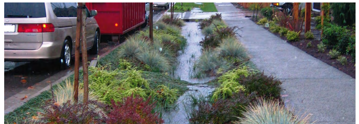
Stormwater Management in the Sidewalk
