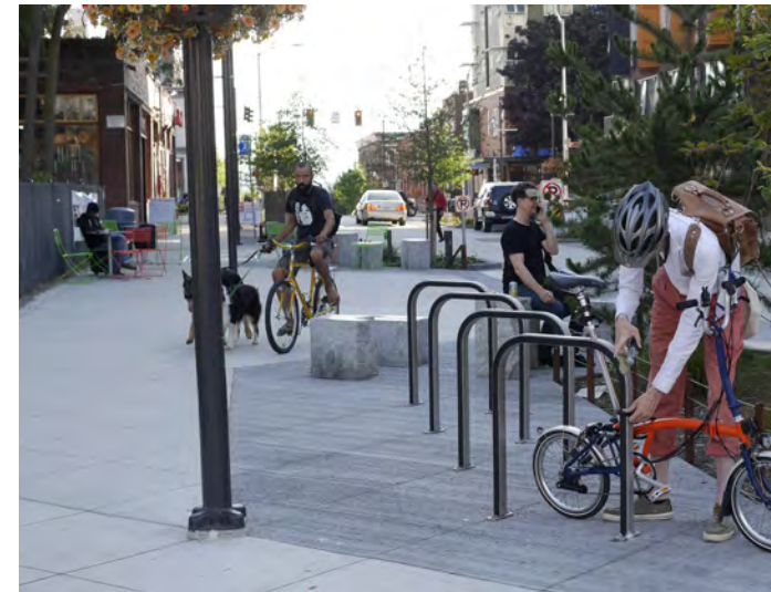
Bicycle Parking Structures
