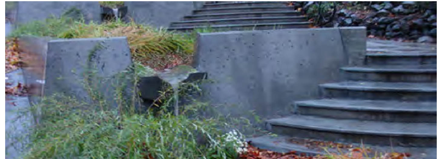
Integrated Stormwater Management Systems
