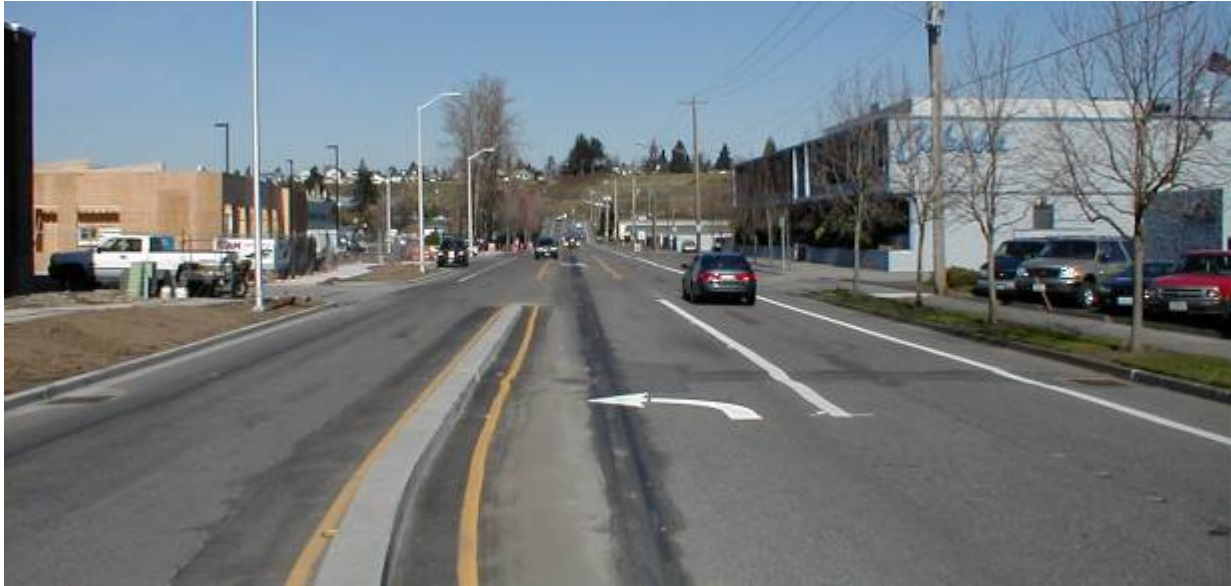
Figure 4 - Grand Boulevard looking north from Columbia House Boulevard - 2008
