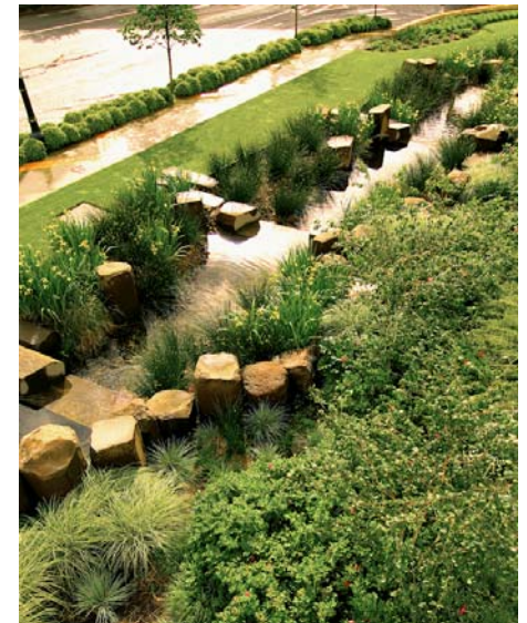
Figure 18. Example of a rain garden/swale.
