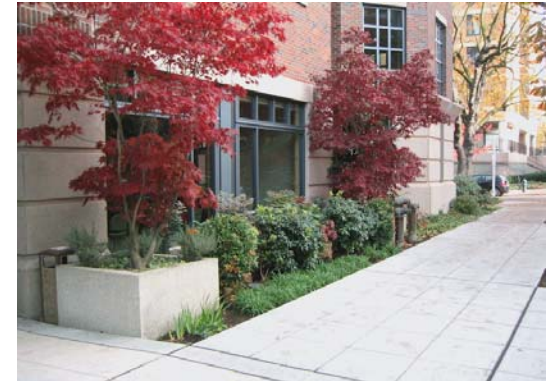
Figure 8. An example of a building along a Mixed-Use Street featuring a landscaped setback. This structure is probably set back less than 10 feet from the sidewalk, but includes attractive landscaping, high quality building materials and transparency, thus it would be a good departure example.
