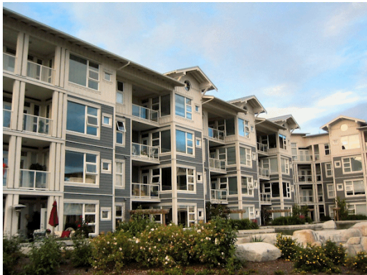
Figure 36. An example of façade articulation at less than 30' intervals.
