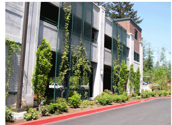
Figure 32. A good example of parking garage screening.
