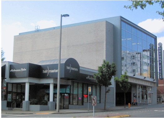
Figure 43. Blank, visible, and plain CMU fire walls like this are prohibited. Such buildings should incorporate patterns of different CMU colors or textures or different materials to add visual interest to such visible firewalls.
