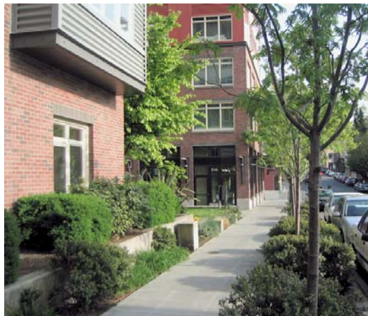
Figure 7. Development along mixed-use streets may have storefronts or modest landscaped setbacks..
