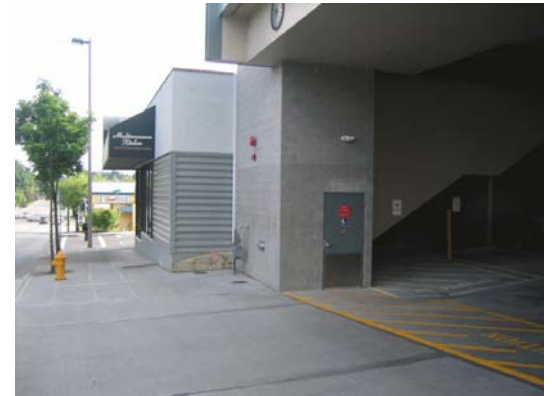
Figure 22. Avoid exposed utility meters like this.
