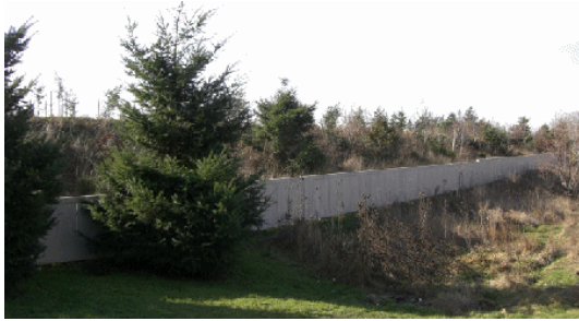
Figure 43. Existing quarry berms may be used to support a trail in conjunction with master planned development as conditions allow.
