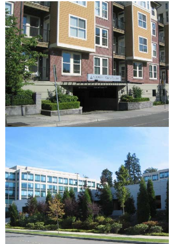
Figure 35. Examples of buildings with structured parking.
