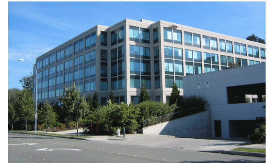
Figure 24. The plan envisions office buildings mixed with retail and multifamily uses in the core areas.
