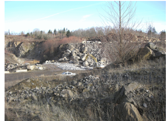
Figure 11. Quarry activities will continue on some portions of the site
