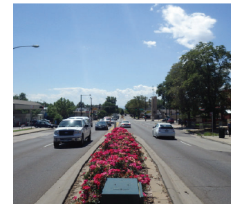
Medians can reduce the frequency and severity of lane departure crashes in urban environments.
