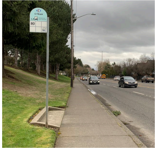
Photograph 2-17. Bus Stop Lacking a Shelter
