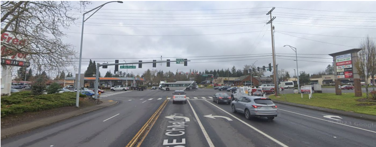
Photograph 2-1. Segment 1: Mill Plain Boulevard Intersection (looking north)
