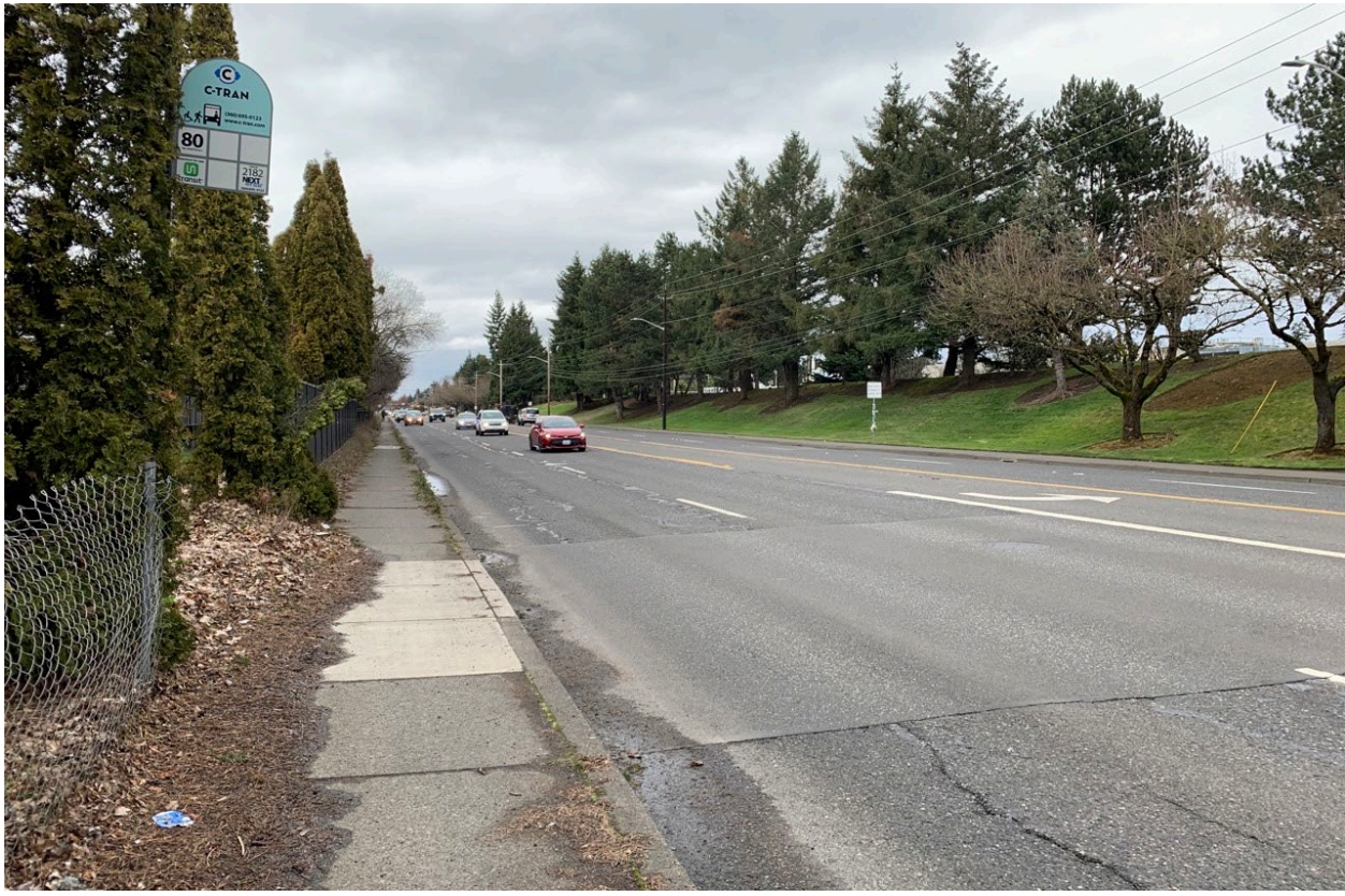
Photograph 2-13. Segment 5: Bus Stop and Vegetation on Sidewalk (looking north)
