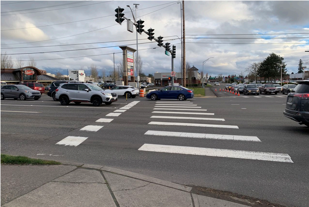
Photograph 2-2. Segment 1: Mill Plain Boulevard Intersection (looking south)
