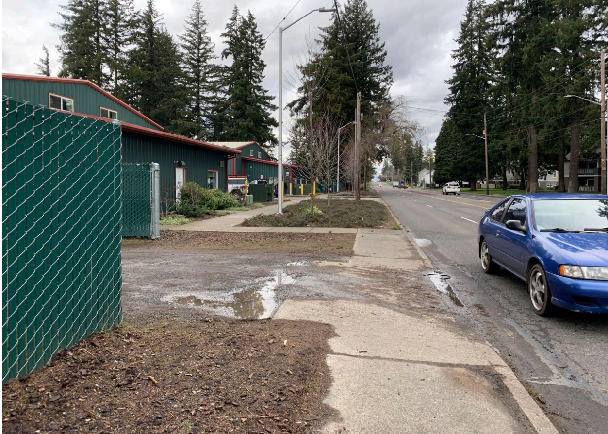
Photograph 2-5. Segment 2: Sharply angled sidewalk configuration (looking north)
