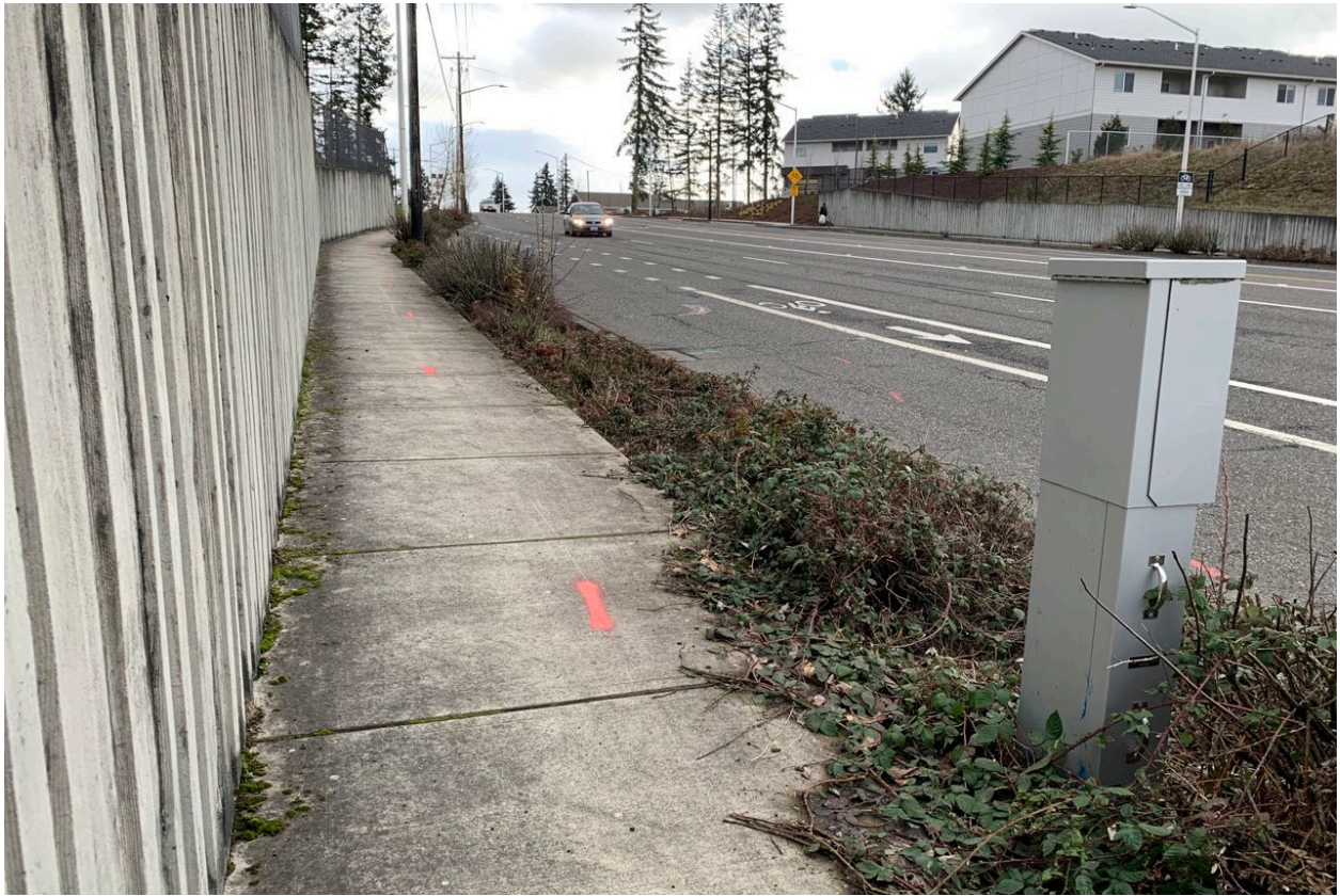
Photograph 2-9. Segment Leaving NE 18th Street Intersection (looking south)
