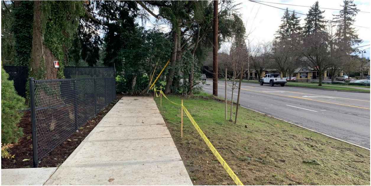
Photograph 2-8. Segment 3: Sidewalk Ends on East Side of Street (looking south)
