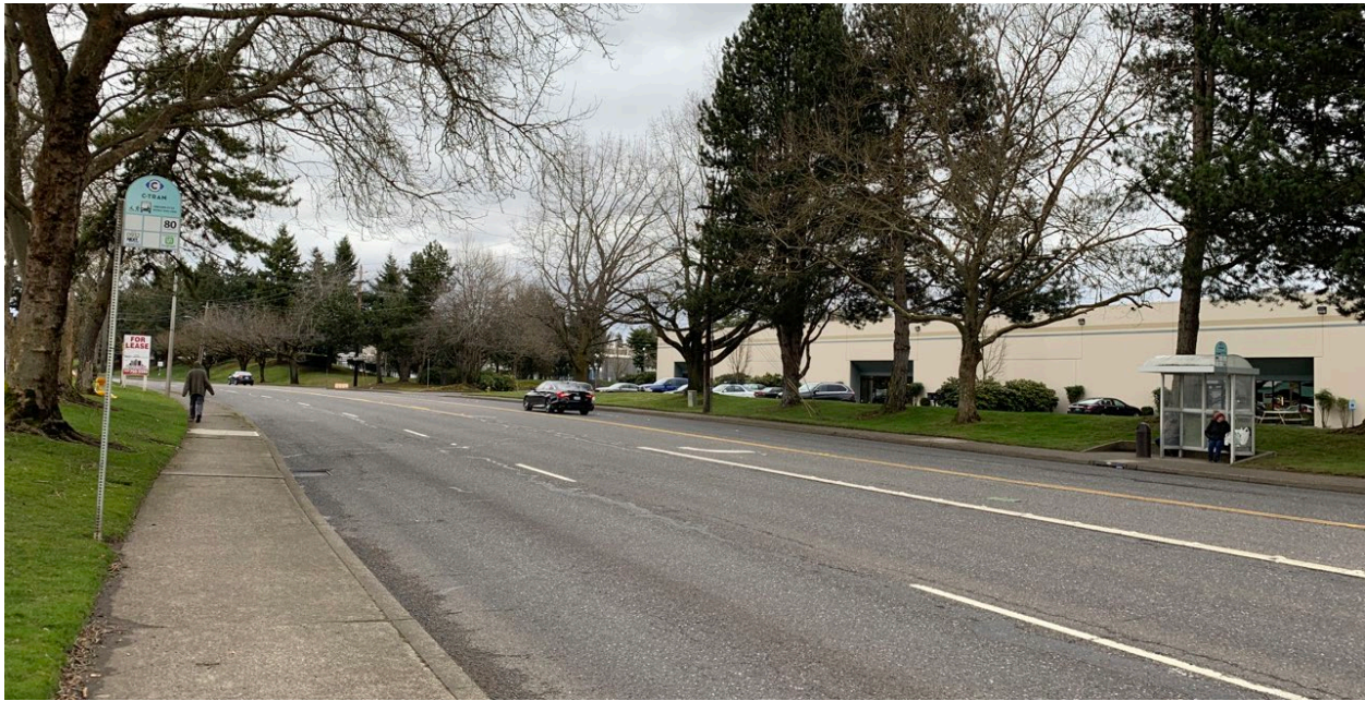
Photograph 2-12. Segment 5 (looking north)
