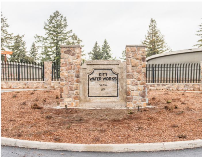
Water Station 1 project increased the security, reliability and performance of the city's water system.
