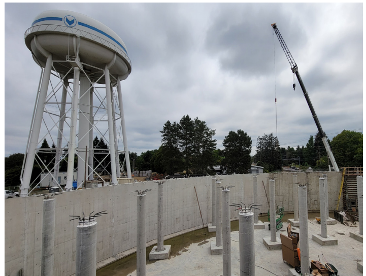
Water Station 5 new reservoir construction.
