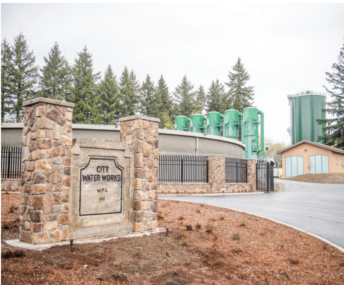
Water Station 1 project increased the security, reliability and performance of the city's water system.
