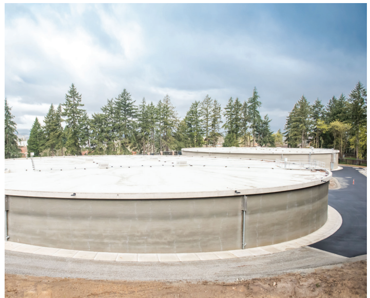
Seismically resilient reservoirs constructed as part of the Water Station 1 Project.
