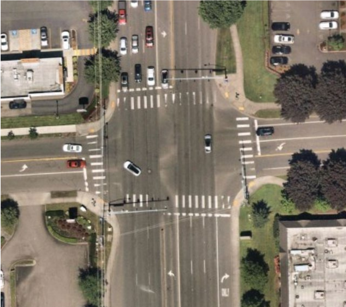
Figure 27 164 th Ave and Tech Center Dr
