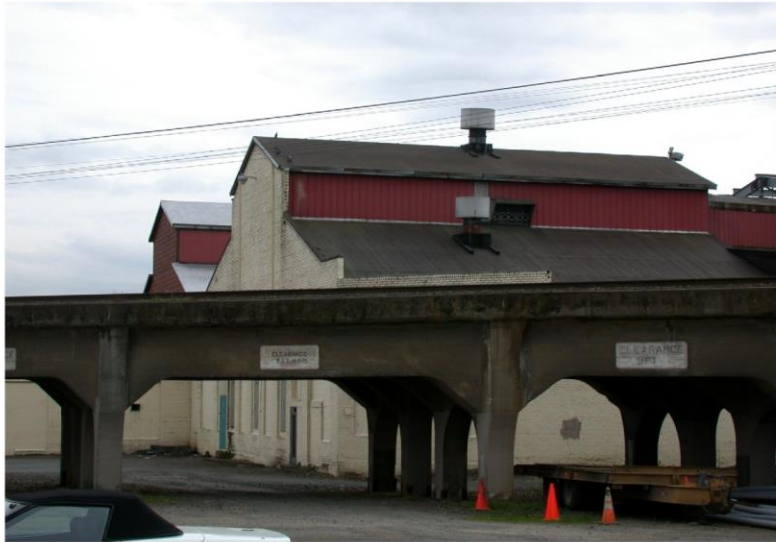
Photo 8-1. The Boise Cascade Complex and the BNSF viaduct are located in the Columbia West Renaissance area. These two resources have not been surveyed. The view is to the southwest.
