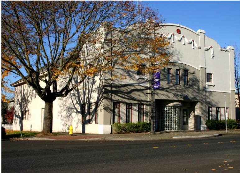
Photo 8-11. The Society Theater (1925) south elevation and east facade. The building is located in the Uptown Village area and is located in the recommended North Main Street Commercial Local Historic Overlay District. The theater has been altered and no longer retains its original interior features or the original entry facade.
