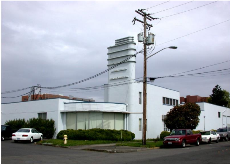
Photo 8-5. Pepsi building (ca. 1935), south facade. The building is located in the Westside Government area and is recommended eligible for the NRHP, WHR, and the CCHR. The view is to the northeast.
