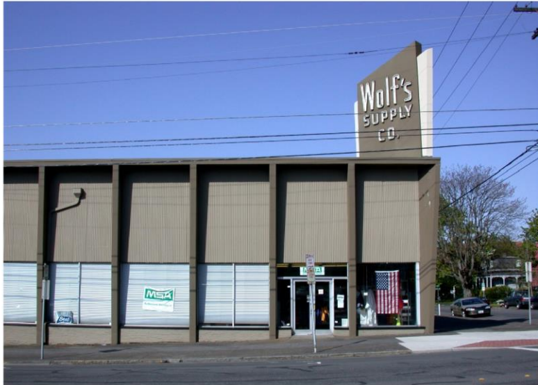
Photo 8-4. The Wolf's Supply Company building (ca. 1951) is one of the first tilt-up concrete buildings in Vancouver. The building is located in the Central Downtown area and is recommended eligible for the NRHP, WHR, and the CCHR. The view is to the west.
