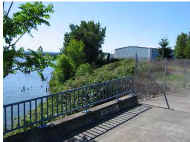
Existing conditions on the waterfront
