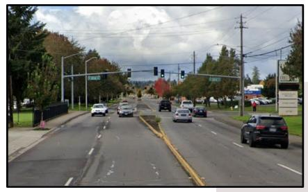
The roadway cross section in this segment varies, and includes a concrete median, intermittent center turn lane, and two long turn pockets for 65<sup>th</sup> Ave and Andresen.
