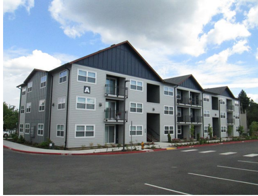
K West Apartments, Fourth Plain & 57 th Avenue, 35 units per acre
