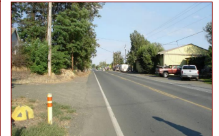
Shoulder bikeways are appropriate along wide roads where vehicles can avoid passing close to bicyclists
