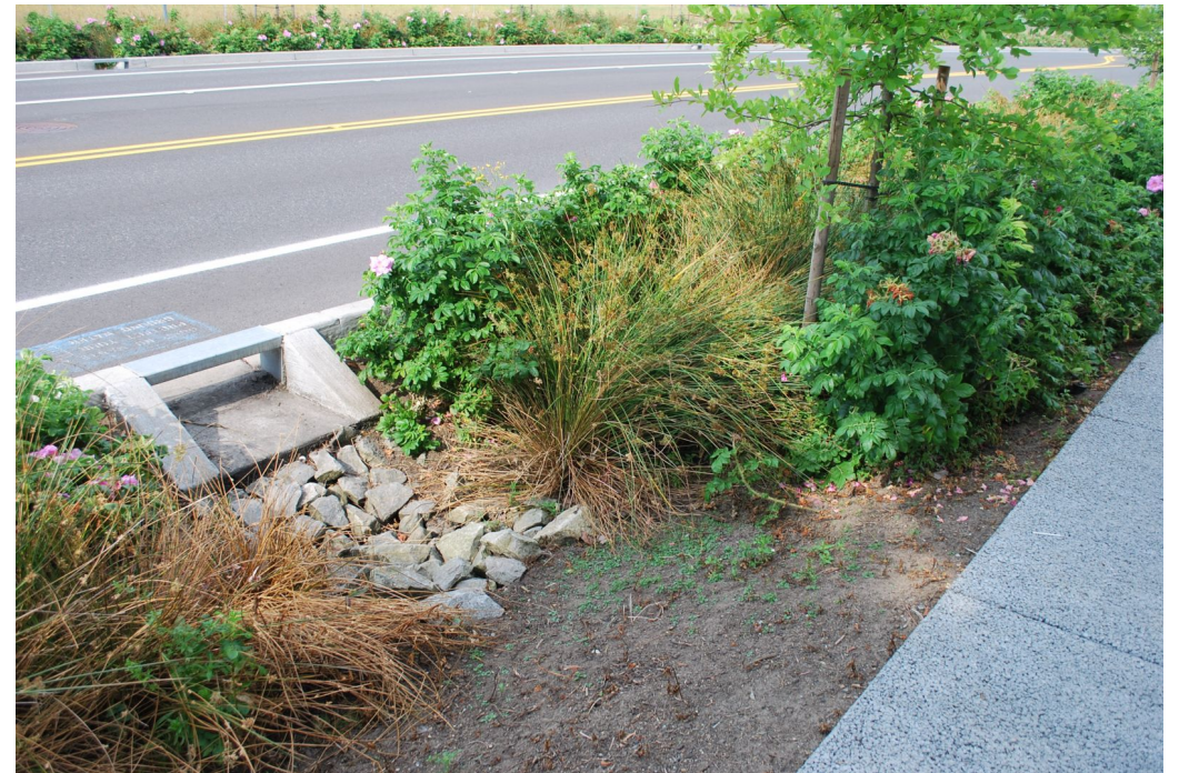
Clark County Green Streets Project on NE 99 th St
