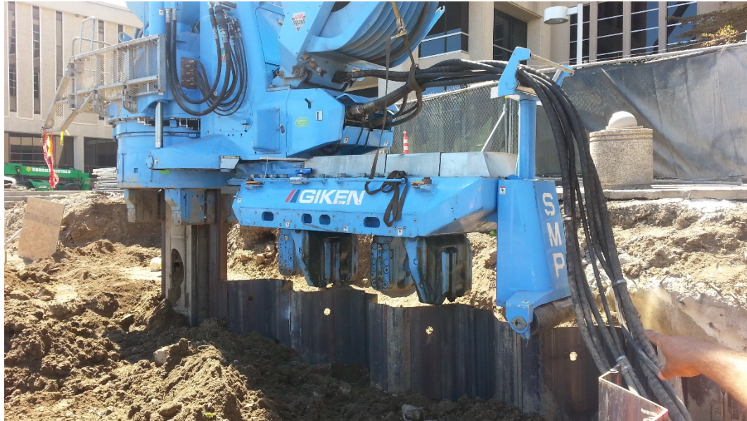
Figure 14. Example of narrow-profile equipment for driving sheet pile
