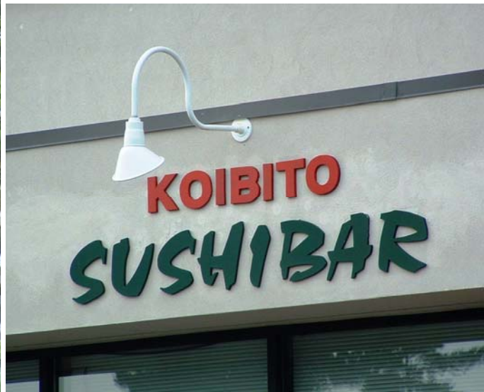
Fully shielded sign light local restaurant (Tumwater Blvd)
