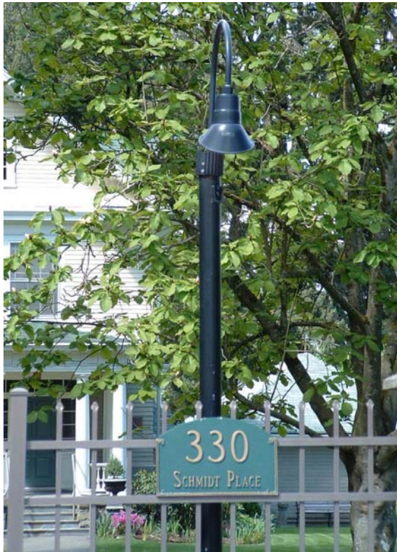
Fully shielded area light at gate to Schmidt House (off Custer)
