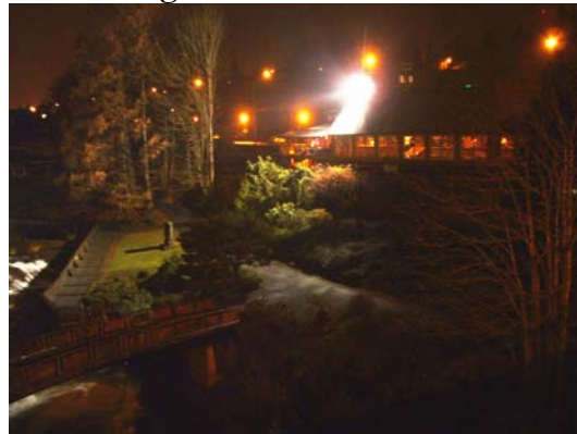
Falls Terrace lights
