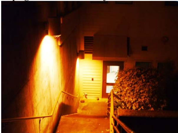
Fully shielded lights on City Hall back steps
