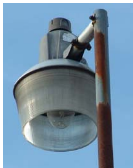
Mercury vapor lamp (Point Tavern)
