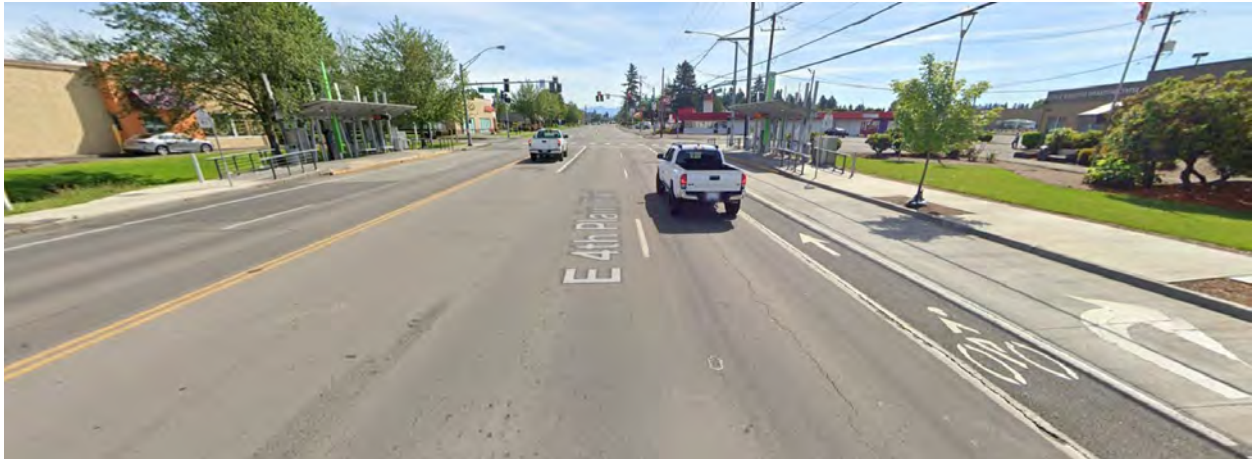
Photograph 5. Dedicated Bike Lanes and The Vine Bus Shelters West of General Anderson Avenue
