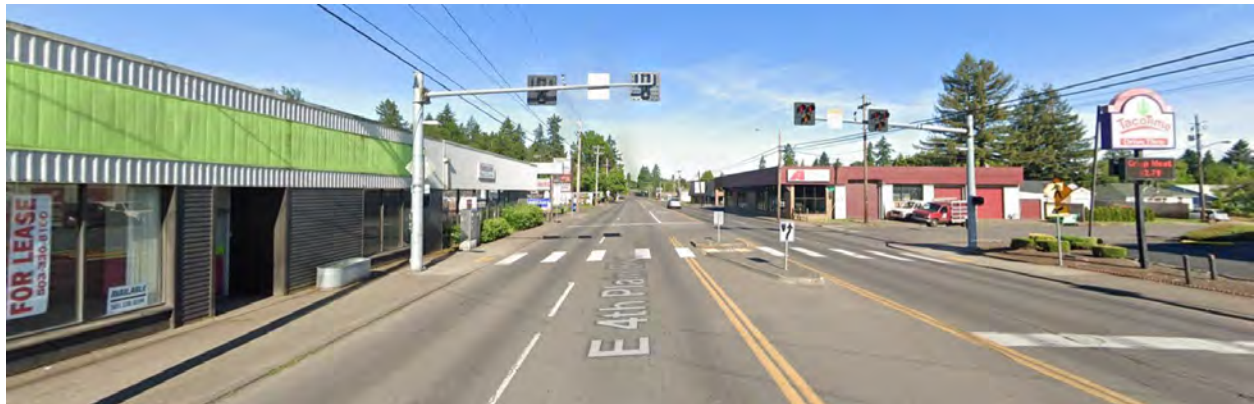
Photograph 4. Enhanced Crossing with Pedestrian Refuge Island on Fourth Plain and Z Street
