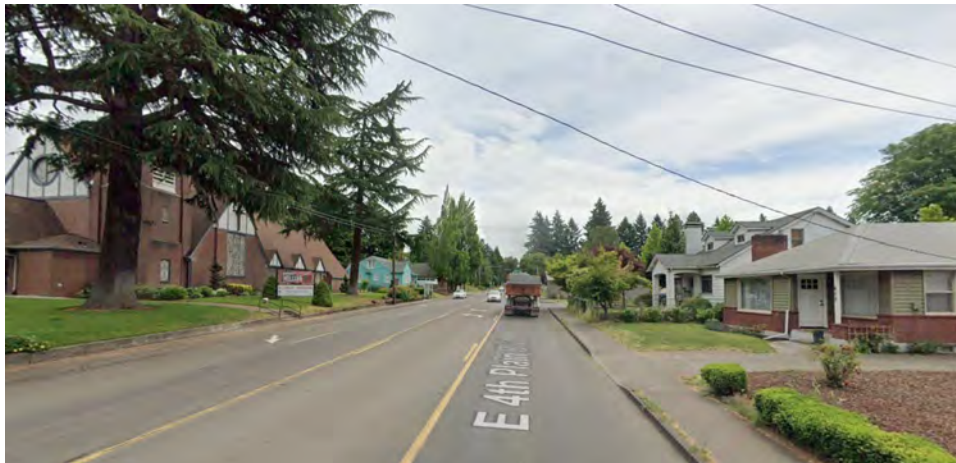
Photograph 1. St. Luke's Episcopal Church and Homes on Fourth Plain Boulevard East of D Street
