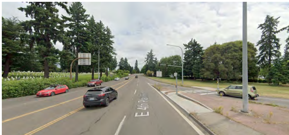
Photograph 2. Fourth Plain Boulevard east of Exit from I-5
