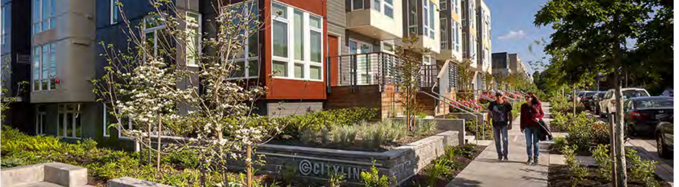
Elevated entryways create building articulation
