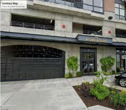
Decorative screening of garage façade
