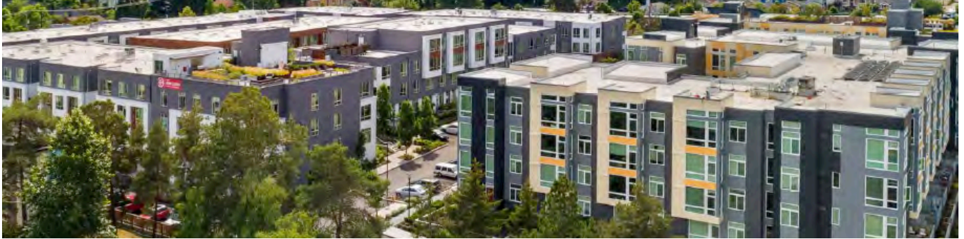
Architectural guidelines create diverse and appealing buildings
