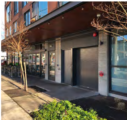
Example of garage parking entrance
