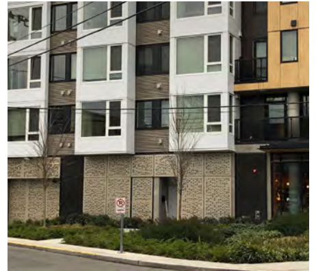
Example of ground level screening
