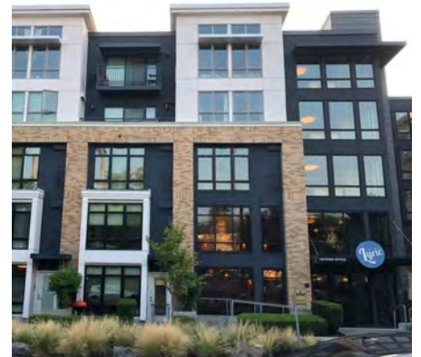
Building with step-down
