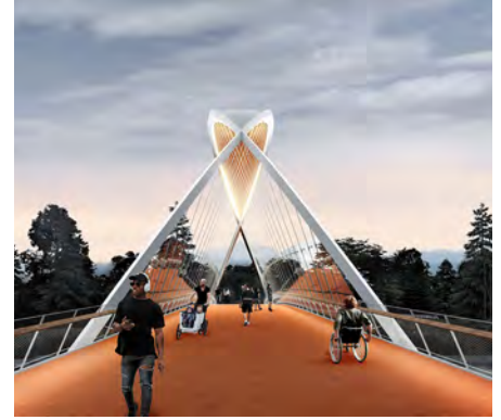
Integrating lighting with structural elements
