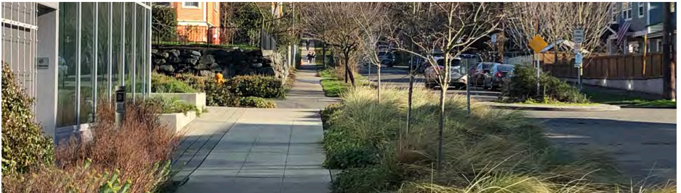
Integrating stormwater management and trees into street design creates attractive and sustainable places
