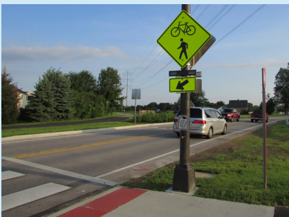
RRFBs used at a trail crossing. Source: LJB
