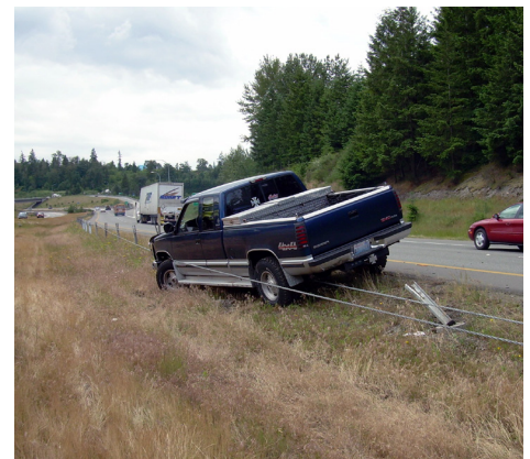
Median cable barrier prevents a potential head-on crash. Source: Washington State DOT
