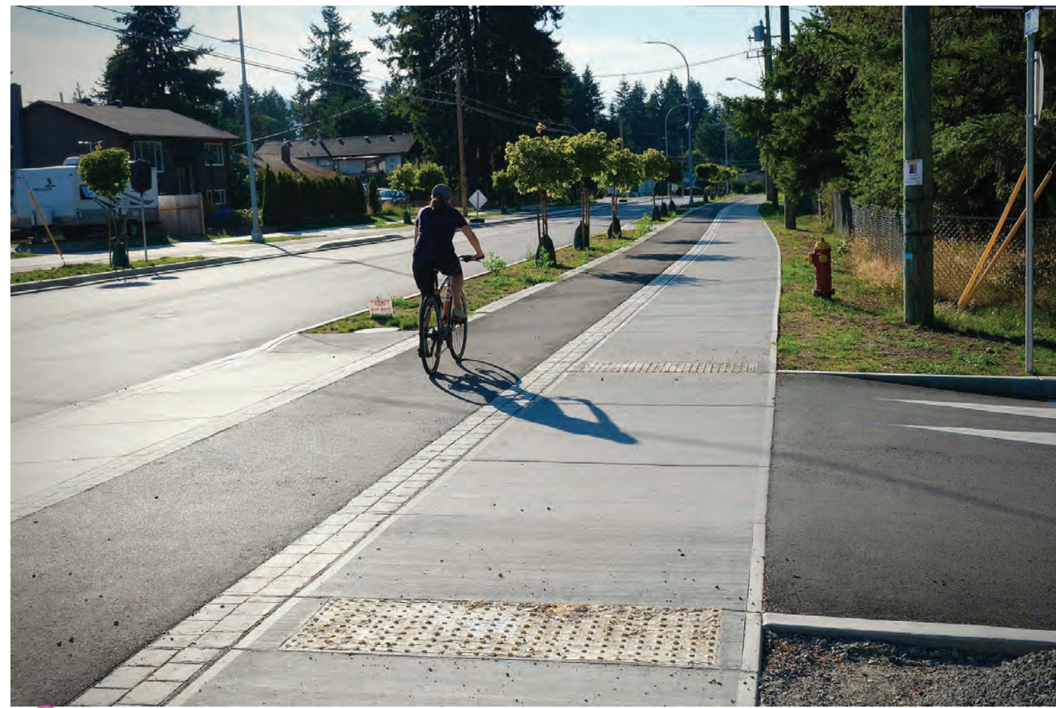
C Street Parking, Curb, Bike Lane, Sidewalk, Street Lights and Stormwater Planters
