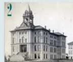
The second courthouse was a three-story brick building that stood in approximately the same location as today's courthouse. Built in late 1883, it went up in flames 7 1/2 years later, destroying a large number of public records. Cost: $44,460 CCHM Collection 01023
