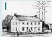
Clark County's first courthouse was a two-story, wood frame structure built in 1855 on West Reserve Street, near Fort Vancouver. Cost: $1,000 CCHM Collection 01006
