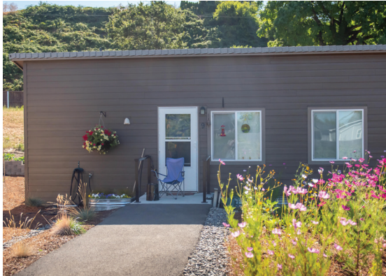
A single unit in Vancouver’s Fruit Valley Terrace, a community providing 21 tiny homes for previously unsheltered residents.
