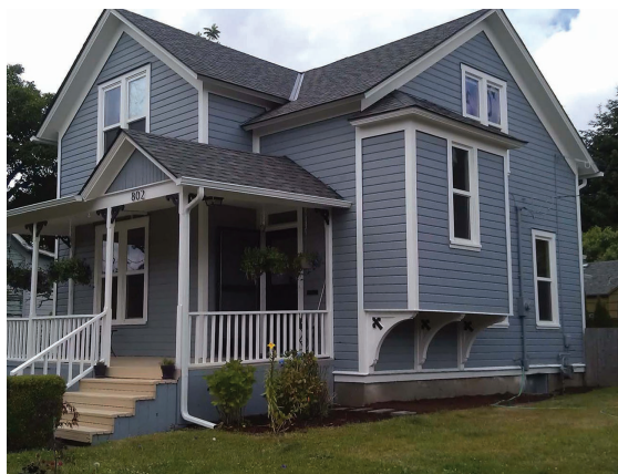
Housing Rehabilitation Program house before (left) and after renovation (right).
