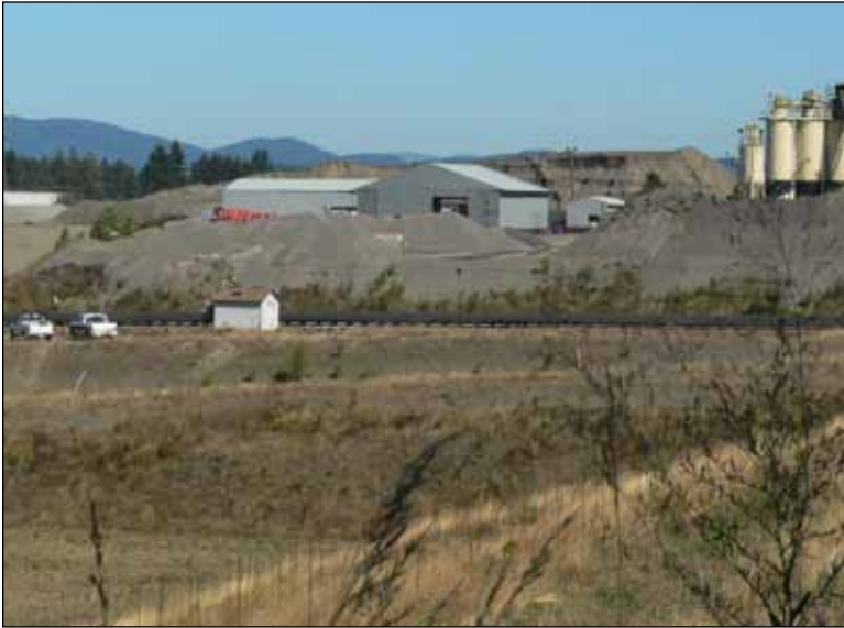
Existing gravel processing
