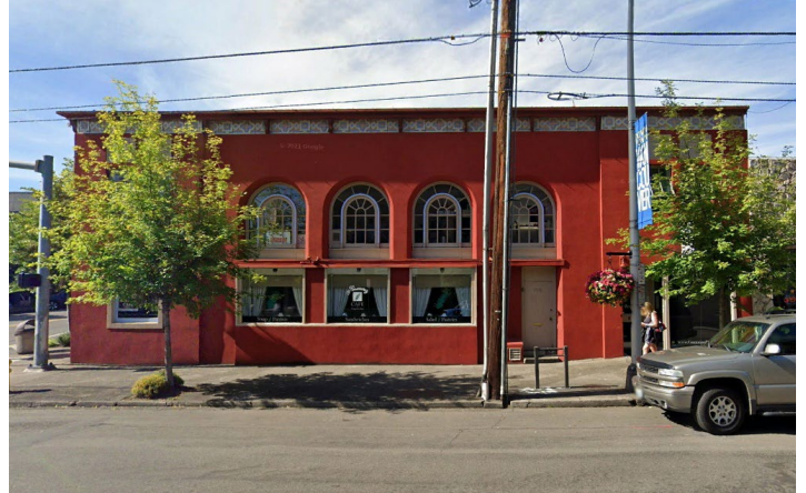
Example of a building with well-articulated ornamentation, artistic fenestration pattern and cornice.
